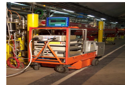
Mobile measurement system TP4&DOC in the LHC tunnel
