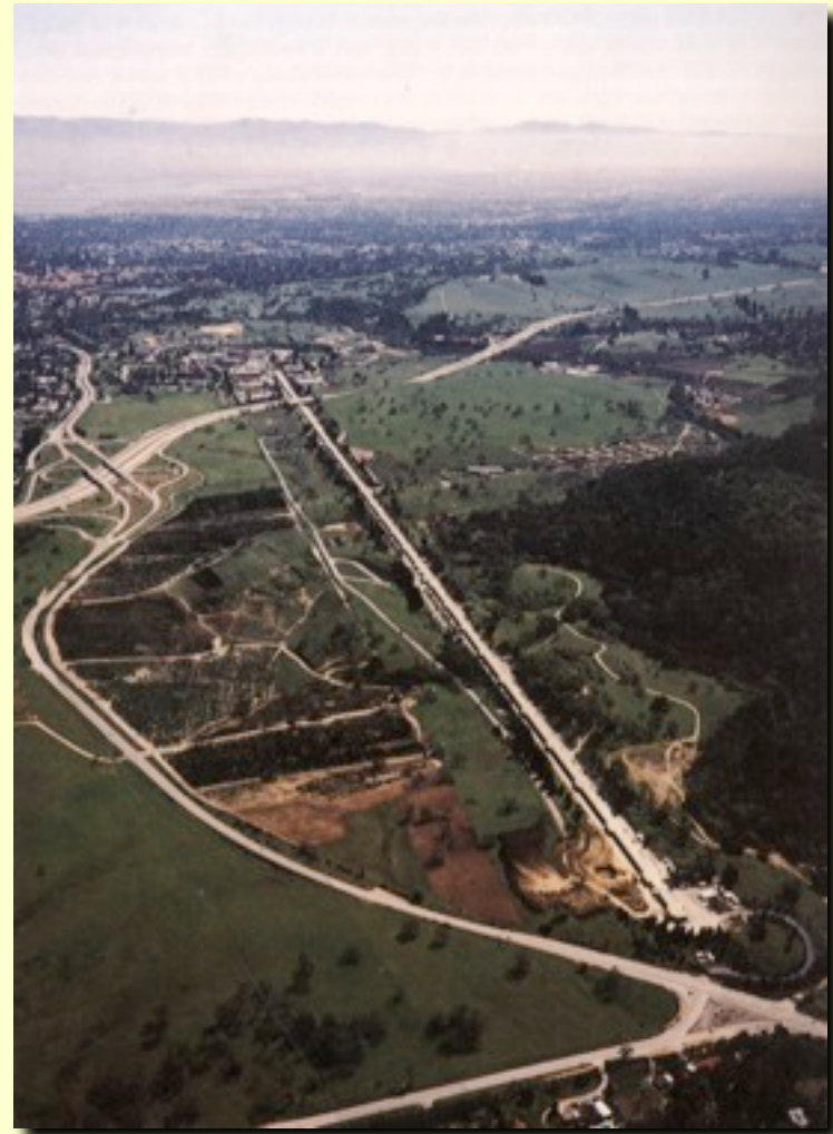
3 km linear accelerator at SLAC (energy 30 GeV)
