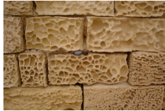
Salt weathering in Gozo, Malta
