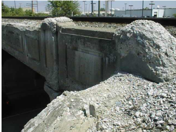
Freeze-thaw scaling of a railroad bridge [Paul Stutzman, NIST]
